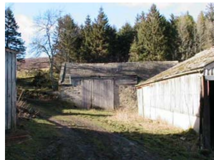
Fig. 13 : access track between the two structures.
